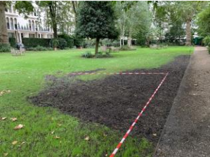
Grass seeding repairs
